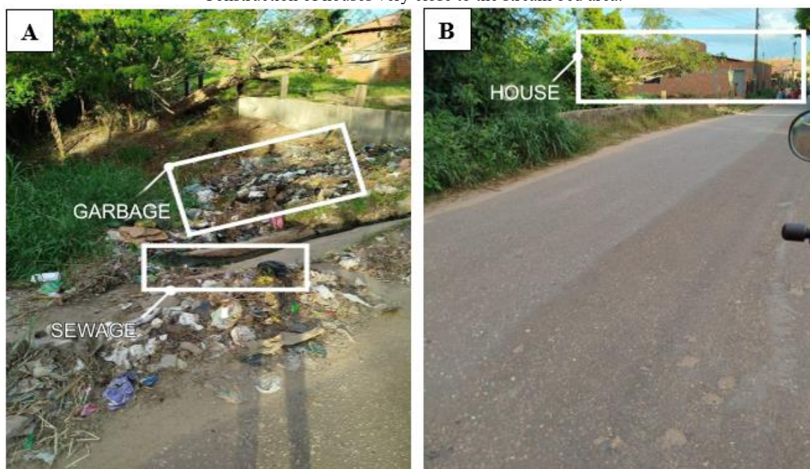
Figure 4 - Section of the Inhamum stream known as Mariinha.. A: Presence of solid waste improperly discarded. B: Construction of houses very close to the stream bed area.
