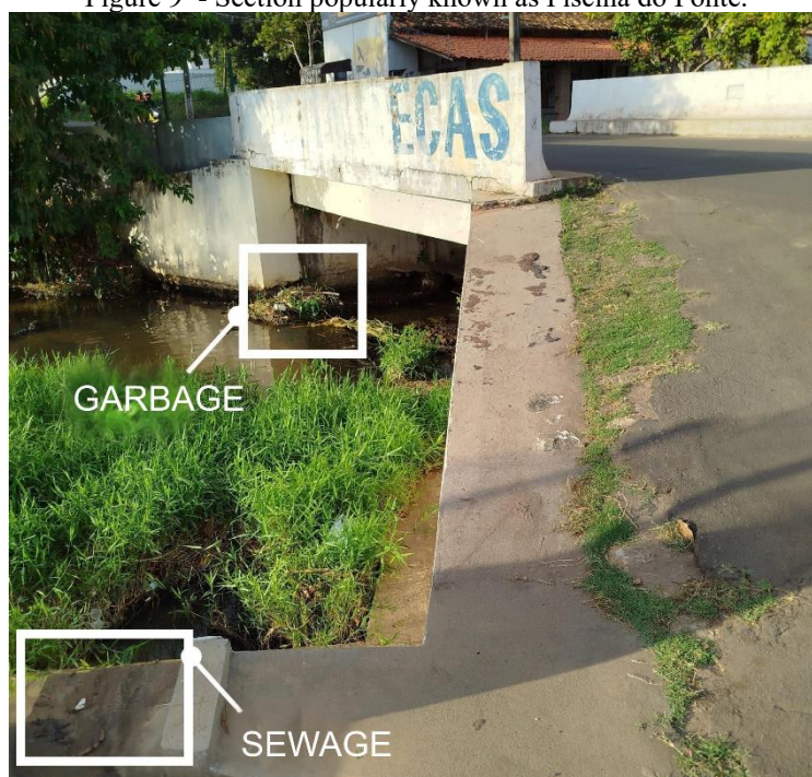
Figure 9 - Section popularly known as Piscina do Ponte.
